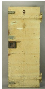
Prison cell door, ca. 1866 H. 186.5 x W. 73.5 x D. 5 cm Painted wood, horizontally placed panels, painted iron, armoured panel and graffiti Donation, 1996 ; inv. AA 1996-0064 © Musée d'art et d'histoire de Genève, photo: B. Jacot-Descombes
